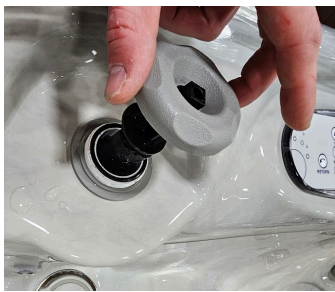
Threaded Cap with Valve Assembly
